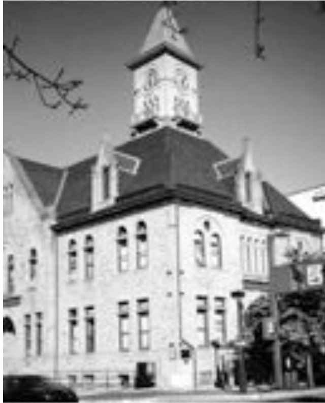
Johnstown's City Hall. The three sets of double markers bracketing the building's corner show the high water marks for the 1889, 1936 and 1977 floods (from top).
